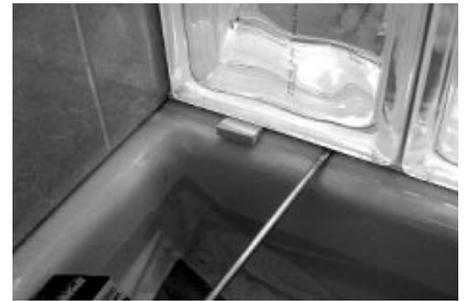
**2.8** Now, that the first course is installed you will need to level the glass blocks using the wedges provided with the anchors. Place a level on top of the first glass block. If the glass block is not level, carefully slide the tip of a screwdriver (straight tip) under the horizontal spacer until the glass block is level. Next, slide a wedge under the horizontal spacer.
