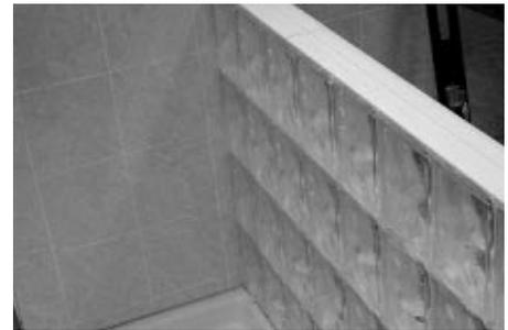
2.13 Check with a level to confirm that the wall is straight, level and plumb as you build. Use a level to check the alignment of the course of glass blocks.
