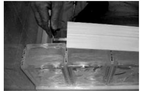
**2.23** Make certain your glass blocks are level from beginning to end. Now you need to assemble the first set of horizontal spacers. Insert a wall anchor in the end of a  $2\frac{3}{8}$  inch horizontal spacer.
