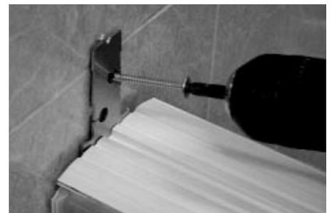
**2.10** Next, apply 1/2 inch beads of sealant to the top of the installed glass blocks behind the raised edge of the glass block faces on both sides of the blocks. Next, install the second horizontal spacer with anchor inserted and push the spacer firmly in place. Install two screws in the anchor (use the screws provided with anchors).
