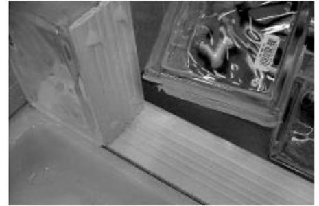
**2.7** Apply 1/2 inch dabs of sealant behind the raised edge of the glass block face 1/2 inch in from the four corners, then press another vertical spacer into place. Apply four 1/2 inch dabs of sealant to the vertical spacer 1/2 inch in from the four-corners. Install the second glass block with sealant side down.
