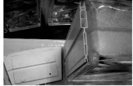
**2.18** Install the first ARQUE® horizontal half spacer with tabs removed. Apply four 1/2 inch dabs of sealant to the side of the last 6 inch x 8 inch glass block, next install the ARQUE® vertical spacer.
