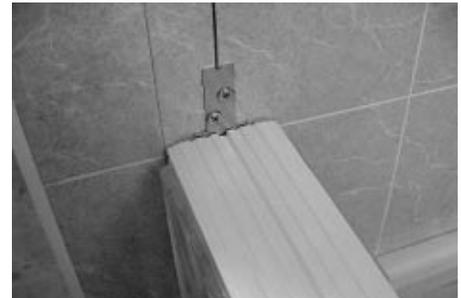
2.27 Now, you will need to draw a plumb line vertically up the wall. Place a four feet level even with the V-notch in the wall anchor and draw a straight, level line on the wall. Install two screws in the anchor (screws provided with anchors). Use this line as a guide when installing the rest of the anchors.
