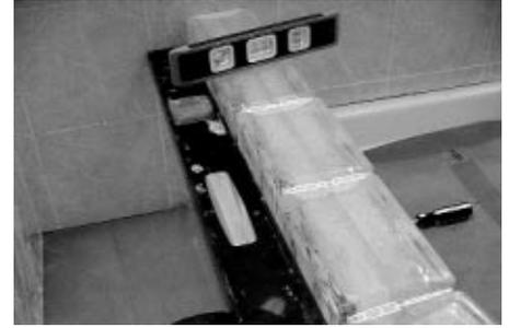
**2.22** Follow the procedures in the straight wall section for leveling each glass block. Use a level to check the alignment of each course of glass blocks.
