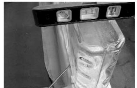
**2.9** Level all the glass blocks. Be sure to slide the wedges between the horizontal spacers and shower base not between the glass block and the horizontal spacer.
