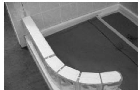
**2.25** Adjust the spacers to fit firmly on top of each glass block.
