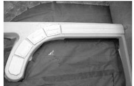
2.16 Install one 6 inch x 8 inch EndBlock™ Finishing Unit after the last ARQUE® vertical spacer. Carefully adjust these blocks to fit the curb and then carefully remove the glass blocks from the bottom horizontal spacers (do not move the bottom spacers).
