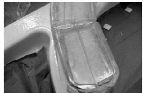
**2.21** Apply four 1/2 inch dabs of sealant to the installed ARQUE® vertical spacer. Next apply a 1/2 inch bead of sealant around the inside perimeter of the finishing unit, then install it on the 4 7/8 inch horizontal spacer.
