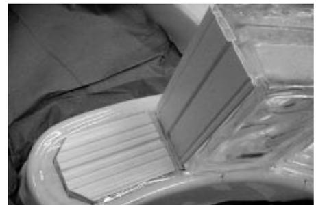
**2.20** Repeat these procedures for the next two ARQUE® glass blocks. Apply four 1/2 inch dabs of sealant to the side of the last installed ARQUE® glass block and apply a 1/2 inch bead of sealant around the inside perimeter of the markings on the curb for the 4 7/8 inch horizontal. Install the ARQUE® vertical spacer and the 4 7/8 inch horizontal spacer.
