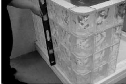
**2.20** Check with a level to confirm that the wall is straight, level and plumb as you build. Use a level to check the alignment of the course of glass blocks.
