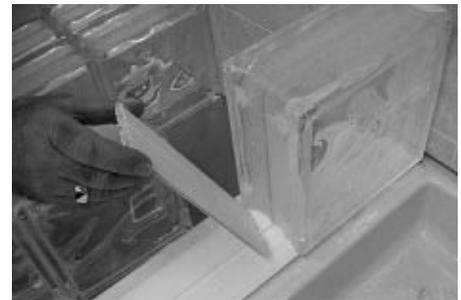
**2.7** Then apply  $\frac{1}{4}$  inch beads of sealant across the top of the first course of blocks, behind the raised edge of the glass block face on both sides of the blocks. Next, install first block on top of the horizontal spacer with the beads of sealant down, push the block firmly against the wall and the base.
