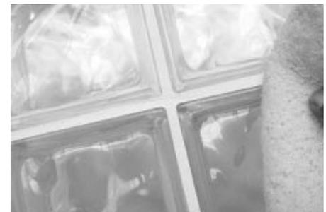
Allow grout to firm up in the joints approximately 5 to 10 minutes, and begin cleaning process. Use a clean tile grout sponge and clean, cool water. Dampen sponge and wring- out as much water as possible. Excessive water during cleanup will weaken grout. Work sponge diagonally to pick up excess grout on surface of blocks. Run sponge lightly through joints to ensure joints are even.
