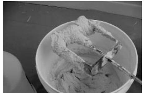
Gradually add half the bag of ProVantage Grout powder while slowly mixing. Use a low-speed mixer. Mix thoroughly to a smooth, homogeneous consistency.
