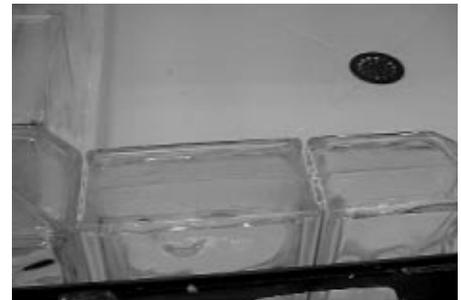
2.14 Use a level to check the alignment and to adjust the first course of glass blocks on the curb.
