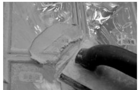
**Begin application of grout:** Starting at the top of the glass block wall, apply grout to the joints of glass blocks by moving the rubber float diagonally on a 45° angle across the joints. This is the best application method to fill the joints with grout. Pack material into joints with float until full. Be carefully not to move glass blocks while grouting since wall might still be flexible prior to grout cure.
