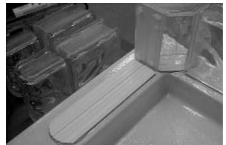
**2.11** Apply four 1/2 inch dabs of sealant to the flat spacer. Remove the 12 7/8 inch horizontal spacer from the curb and apply a 1/4 inch bead of sealant around the inside perimeter of the spacer marking on the curb. Reinstall the 12 7/8 inch horizontal spacer on curb inside the marking.
