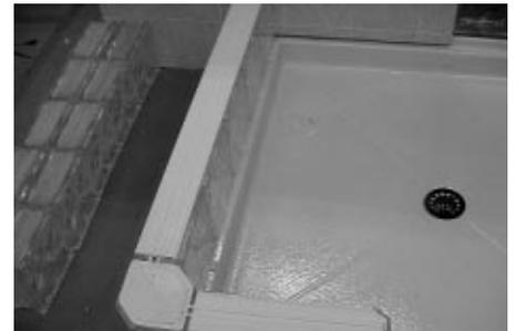
2.17 Place assembled spacers on top of first course of glass blocks and adjust them to fit firmly on the glass blocks. Remove the assembled spacers and apply 1/4 inch beads of sealant across the top of the first course of blocks circling the perimeter of the HEDRON® glass block and the finishing unit. Reinstall the assembled spacers, make certain the spacers are fitting firmly on the glass blocks.
