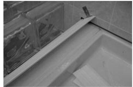
**2.5** Now, let's build the walls. Apply  $\frac{1}{4}$  inch beads of sealant on top of the curb  $\frac{1}{4}$  inch inside the lines on both sides where the horizontal spacer was positioned. Then reinstall the horizontal spacer, pressing it down into the sealant. (Do not secure with screws).
