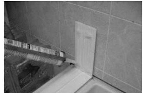
**2.6** Apply four  $\frac{1}{2}$  inch dabs of sealant to the first vertical spacer  $\frac{1}{2}$  inch in from the 4 corners. Press the spacer into place over the anchor. Apply 4 dabs of sealant to the other side of the first vertical spacer.
