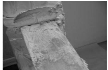
**IMPORTANT:** Use the margin trowel to thoroughly pack the grout in the joints of the EndBlock Finish Units. Apply all the mixed grout before begin the cleaning process.
