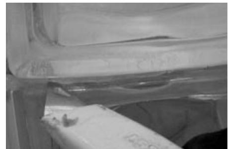
Before beginning the application of the grout, inspect the glass block joints and remove any excess sealant from the vertical and horizontal joints with a utility knife.
