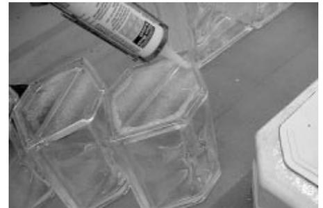
**2.9** Next, remove the HEDRON® half spacer from the curb and apply a 1/4 inch bead of sealant around the inside perimeter of the marking on the curb for the HEDRON® glass block. Reinstall the half spacer, next, apply a 1/4 inch bead of sealant around the top perimeter of the HEDRON® block.
