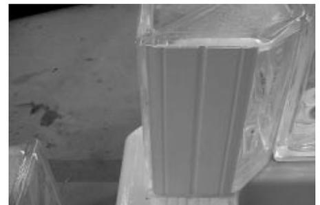
**2.10** Next, install the HEDRON® glass block on top of the half spacer, sealant side down, and push the block firmly into place. Apply four 1/2 inch dabs of sealant to the HEDRON® glass block and install another flat spacer with the flat side against the HEDRON® glass block.
