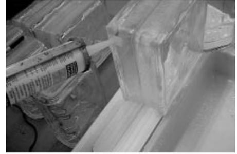
2.12 Next, apply  $\frac{1}{4}$  inch beads of sealant across the top of the 8 inch x 8 inch glass block and round the perimeter of the finishing unit behind the raised edge of the glass block face on both sides of the blocks. Now install the 8 inch x 8 inch glass block on the  $12\frac{7}{8}$  inch horizontal spacer, sealant side down. Now apply  $\frac{1}{2}$  inch dabs of sealant behind the raised edge of the glass block face  $\frac{1}{2}$  inch in from the four corners.
